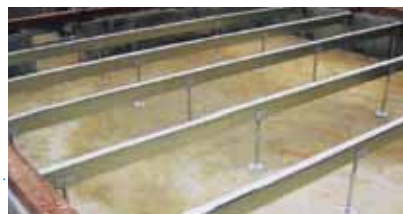
搁栅托梁、短柱
